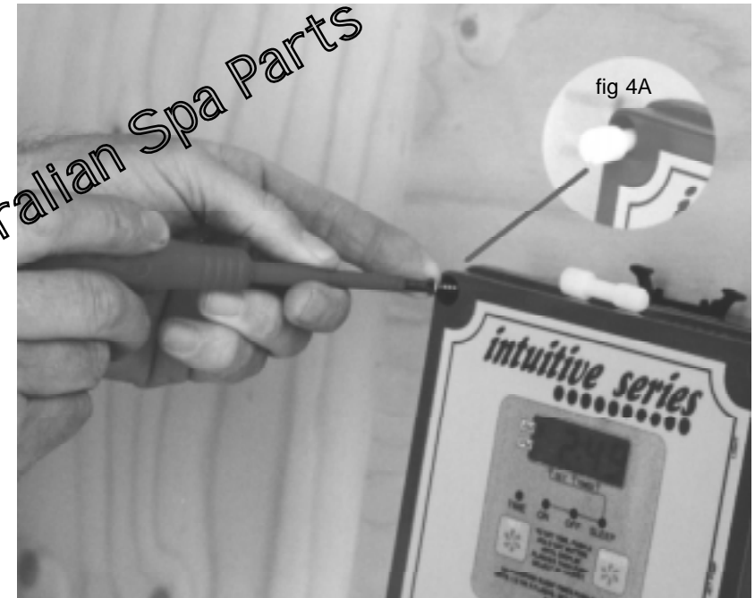
fig 4: Mounting method for control box.
